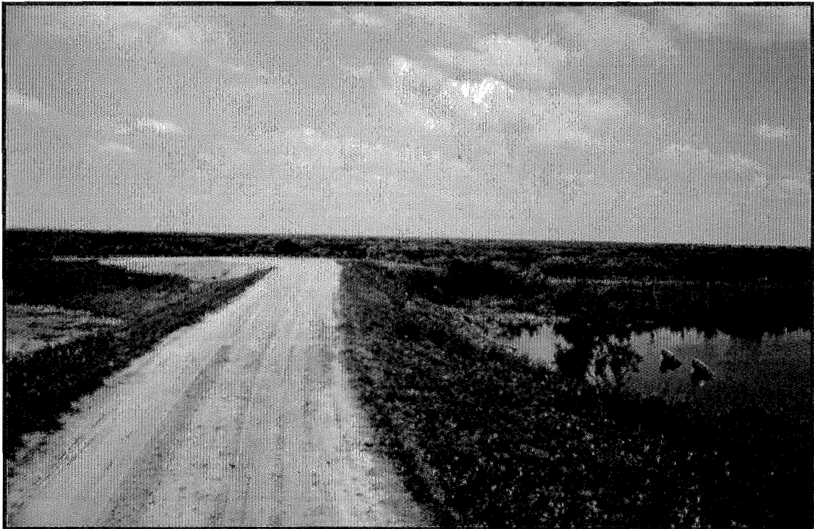
Structure-255, looking south. (Note; only two gates visible in this photo).
