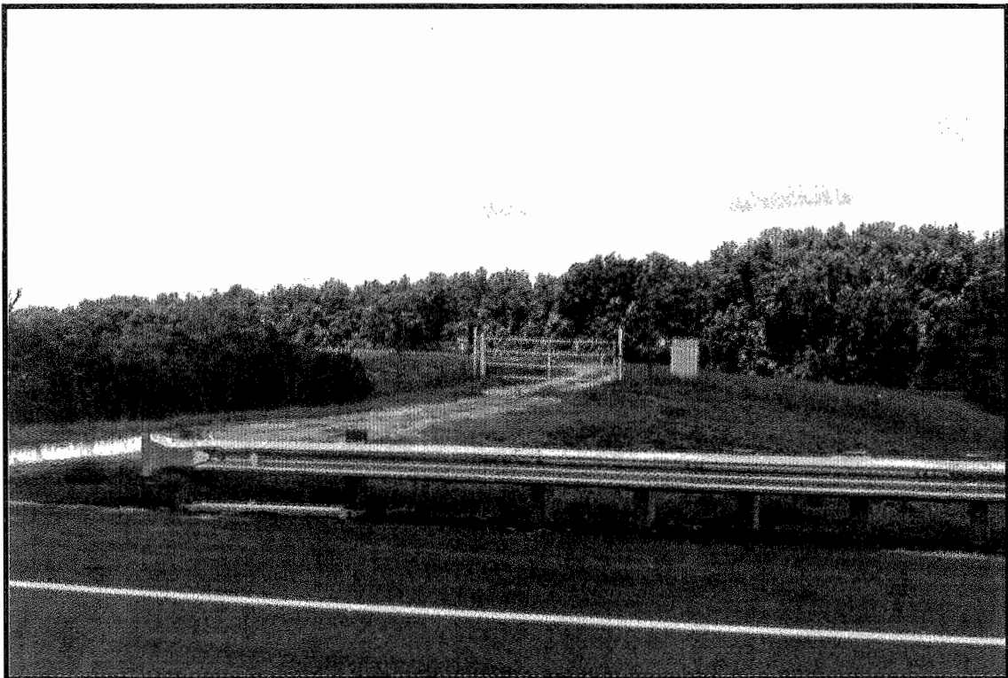
Levee-73-S, looking south at entrance gate off of US-192.
