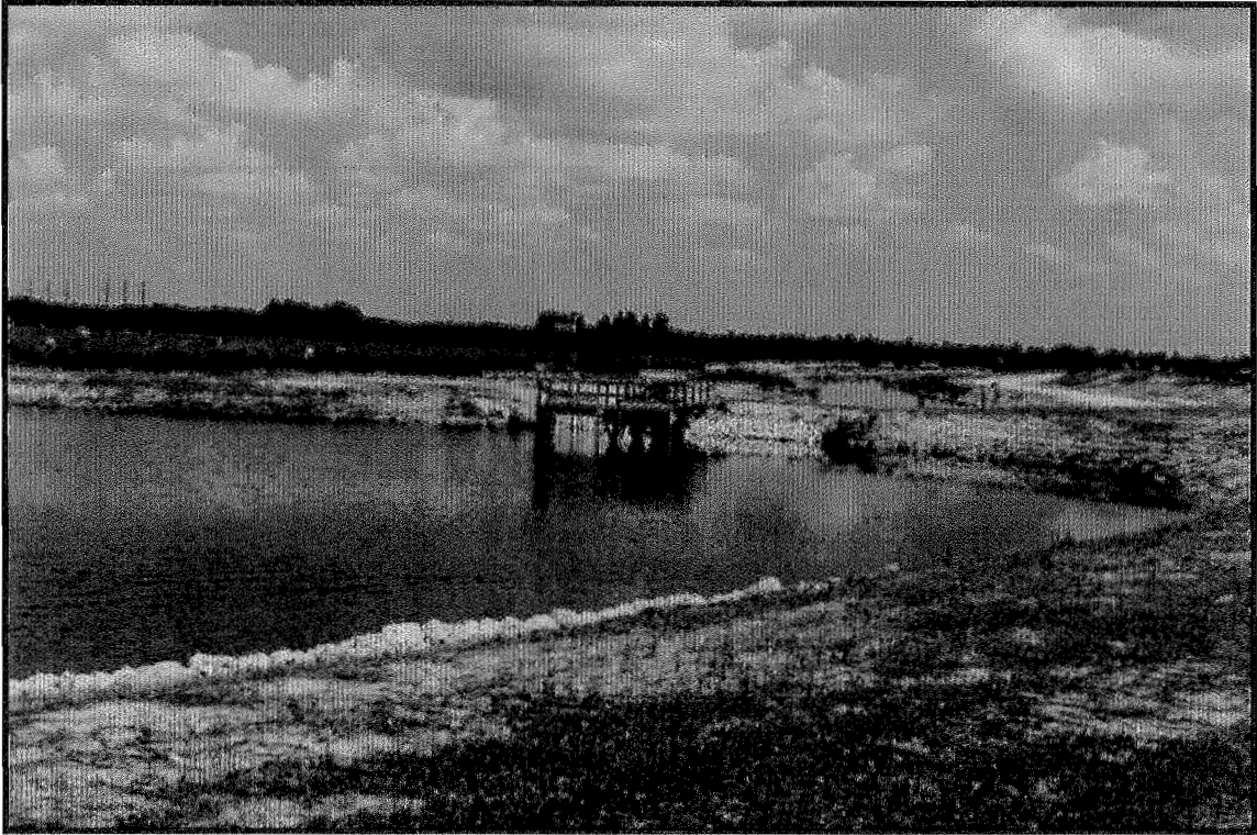
Structure-252-F, looking northwest from S-252-E.
