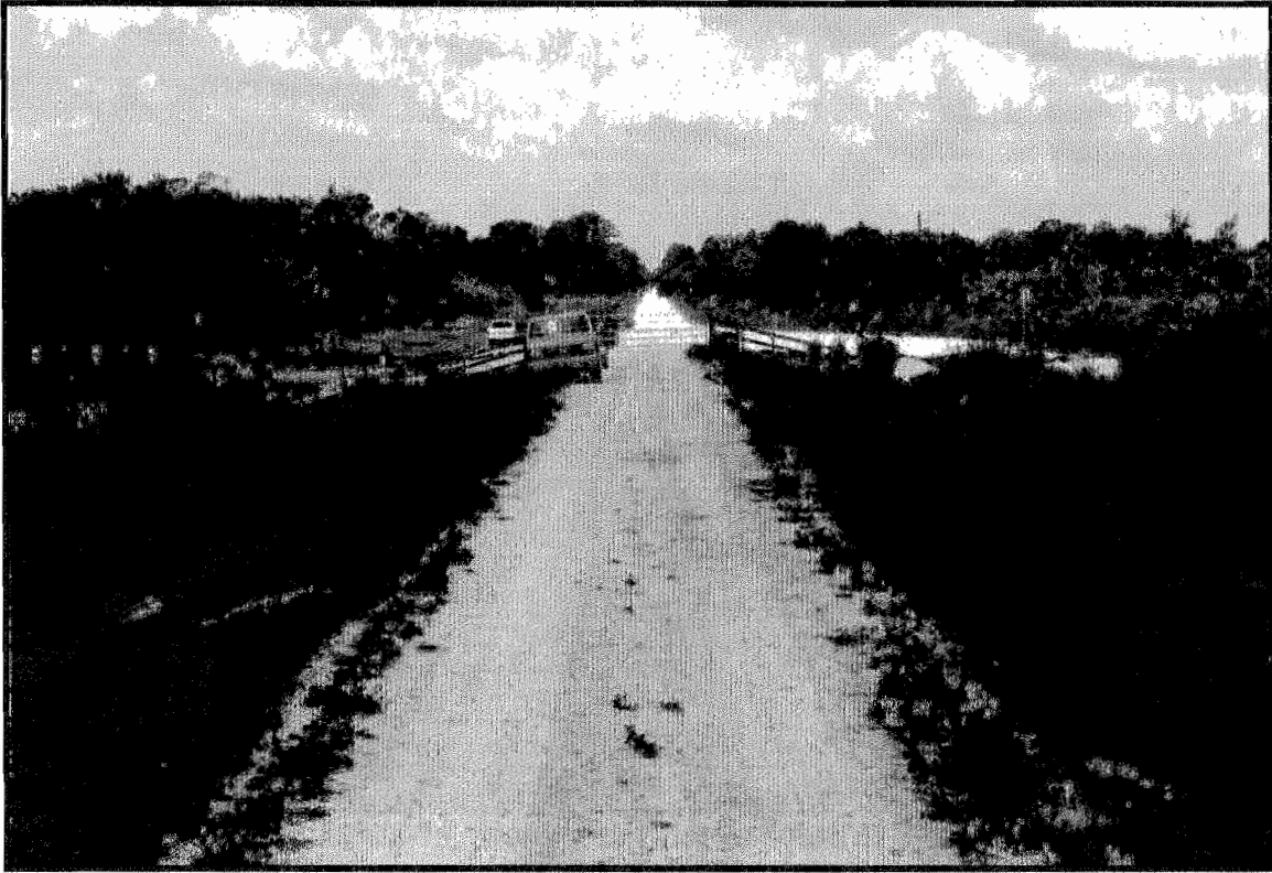
Levee 74-W, looking west across Kenansville Lake Boat Launch.
