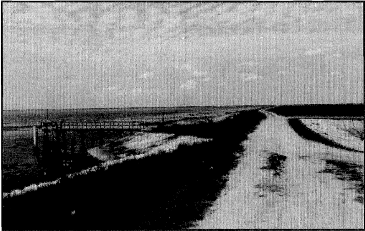
Structure-259, looking north along L-75.
