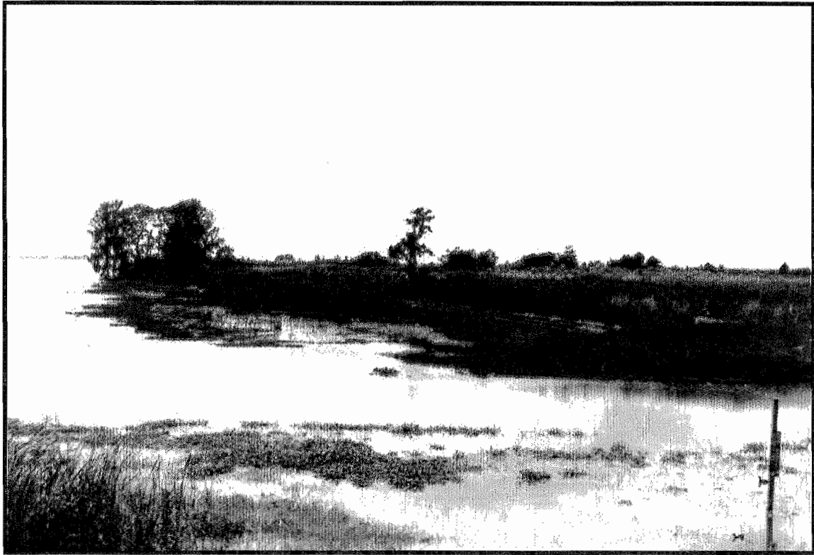
S-254 Weir, looking southwest from L-77-N.
