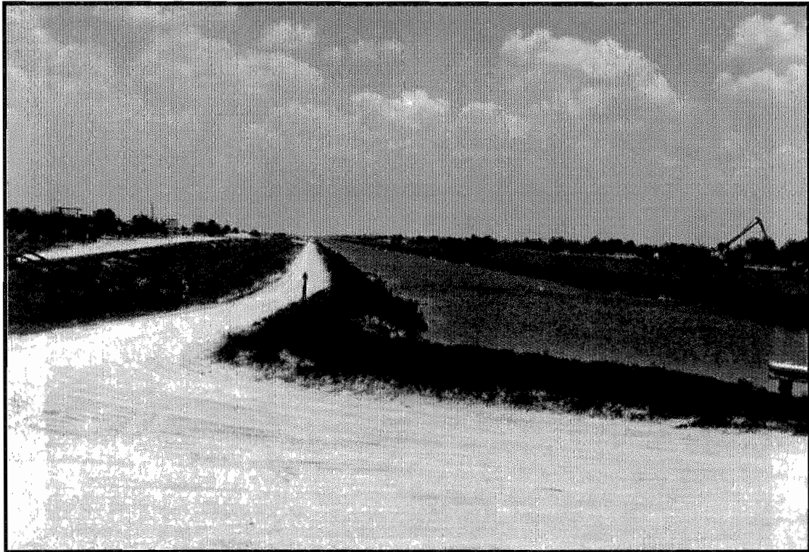
Canal 54, looking east from S-96.
