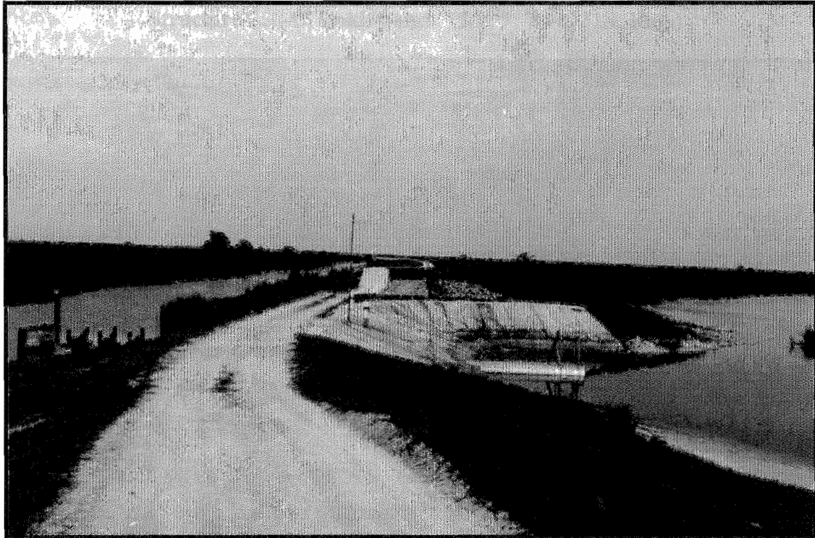
Structure-250-B, looking west. (Sec. 8; Twp. 31S; Rng. 36E)
