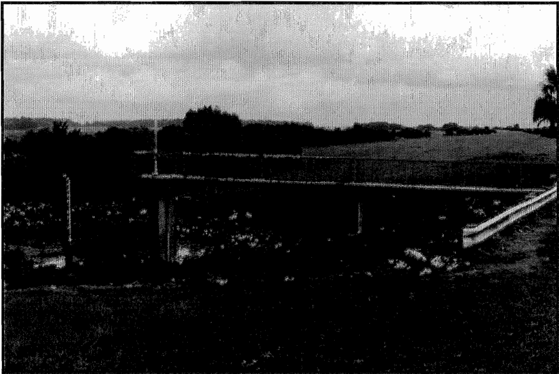
Structure-231, looking north (Cox Creek).
