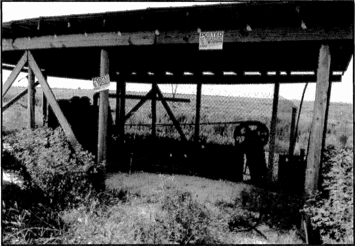
Tucker-East Pump Station, looking south.
