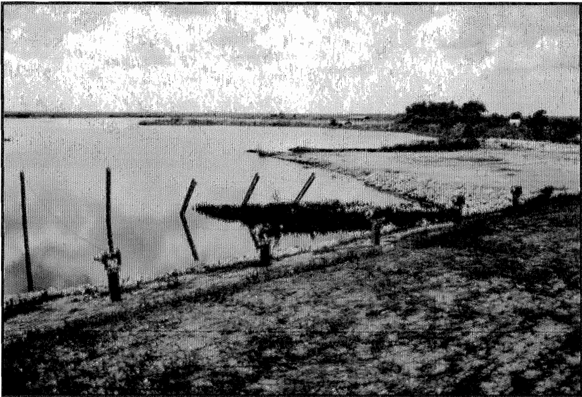
Structure-252-E, looking southeast.
