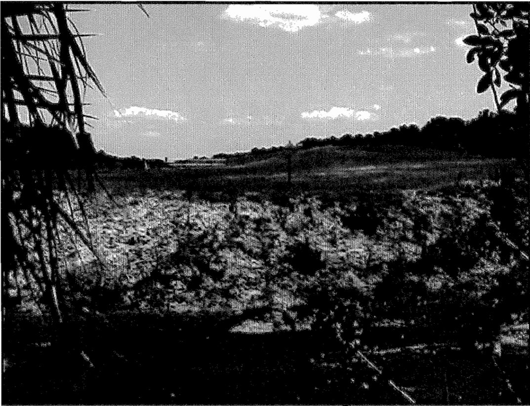
Levee-1, looking east from corner of Canal-1/Canal-2
