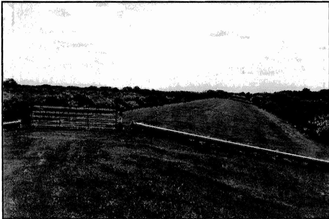
Levee 77-S, looking east near the SR-60 entrance gate.
