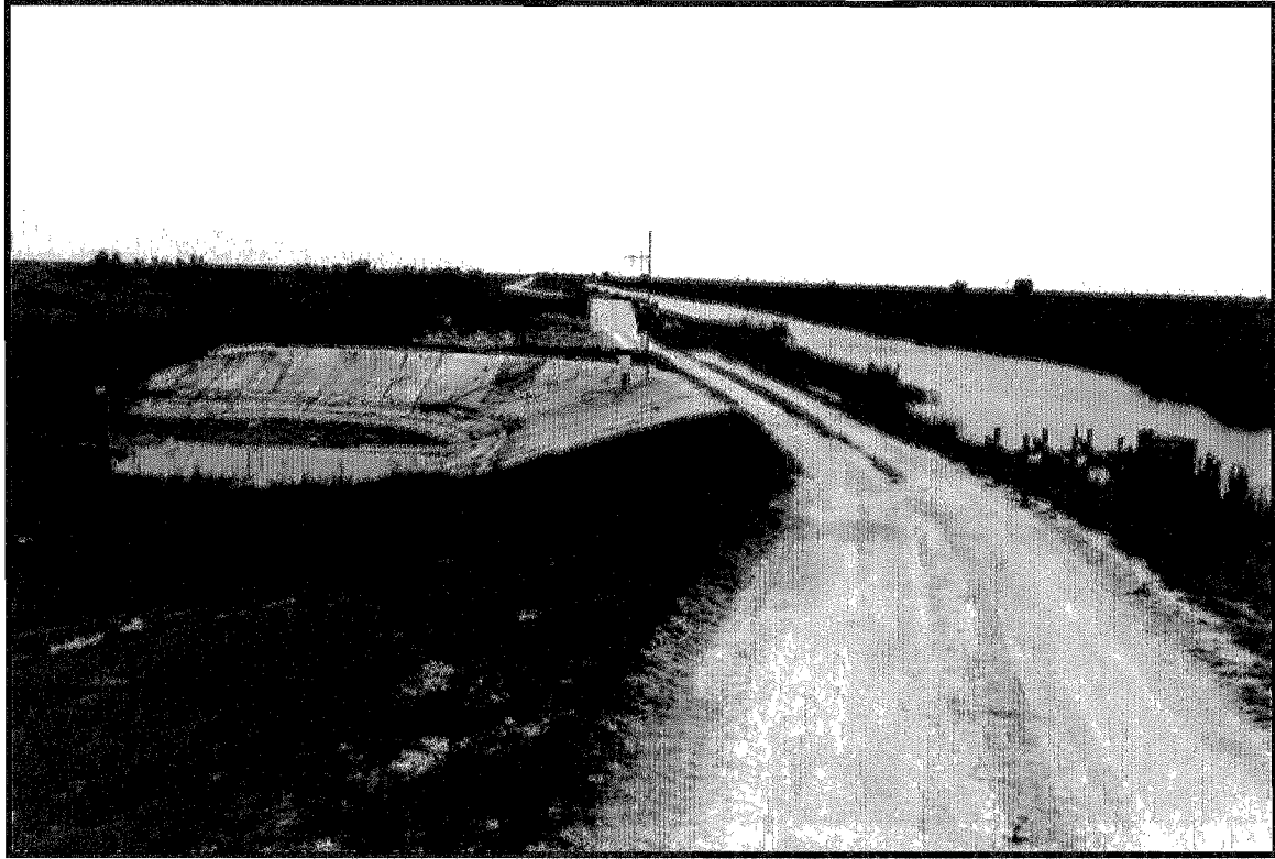
Structure-250-C, looking east. (Sec. 9; Twp. 31S; Rng.)
