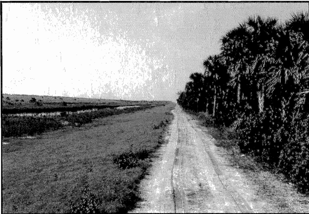
Levee 40, looking south in the Three Forks area.
