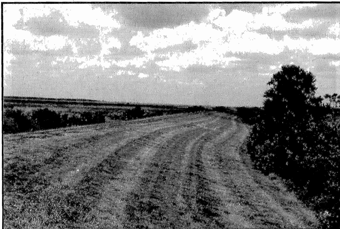
Levee-78, looking west from entrance gate near L-79.
