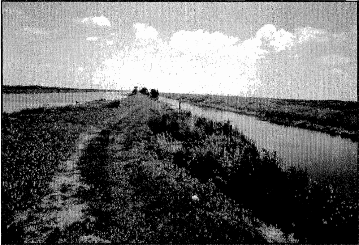
Structure-4, looking south from S-96-D.
