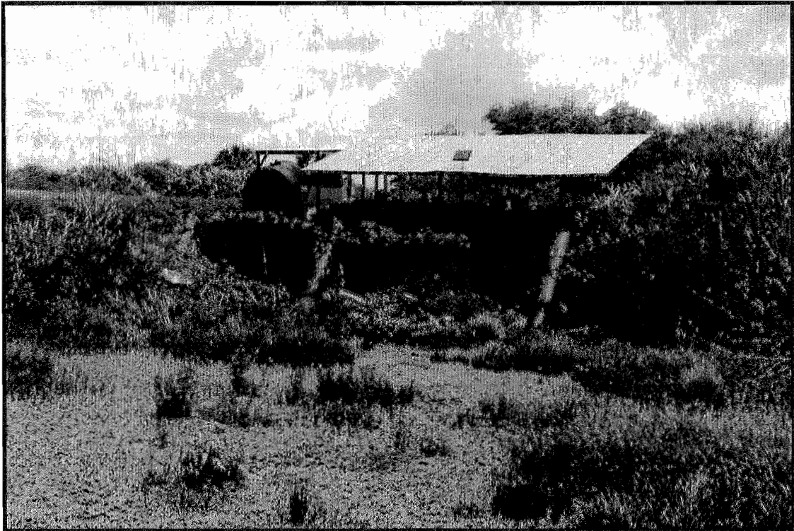
Tucker-West Pump Station
