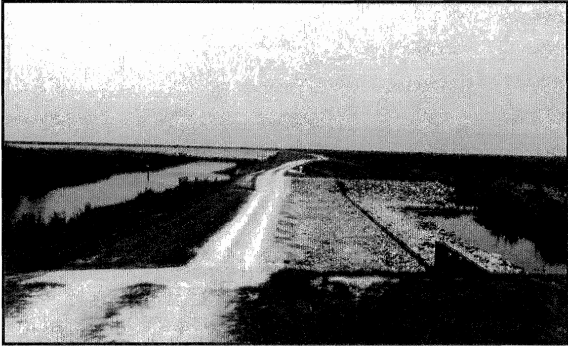
Structure-250-A, looking west. (Sec. 8; Twp. 31S; Rng. 36E)
