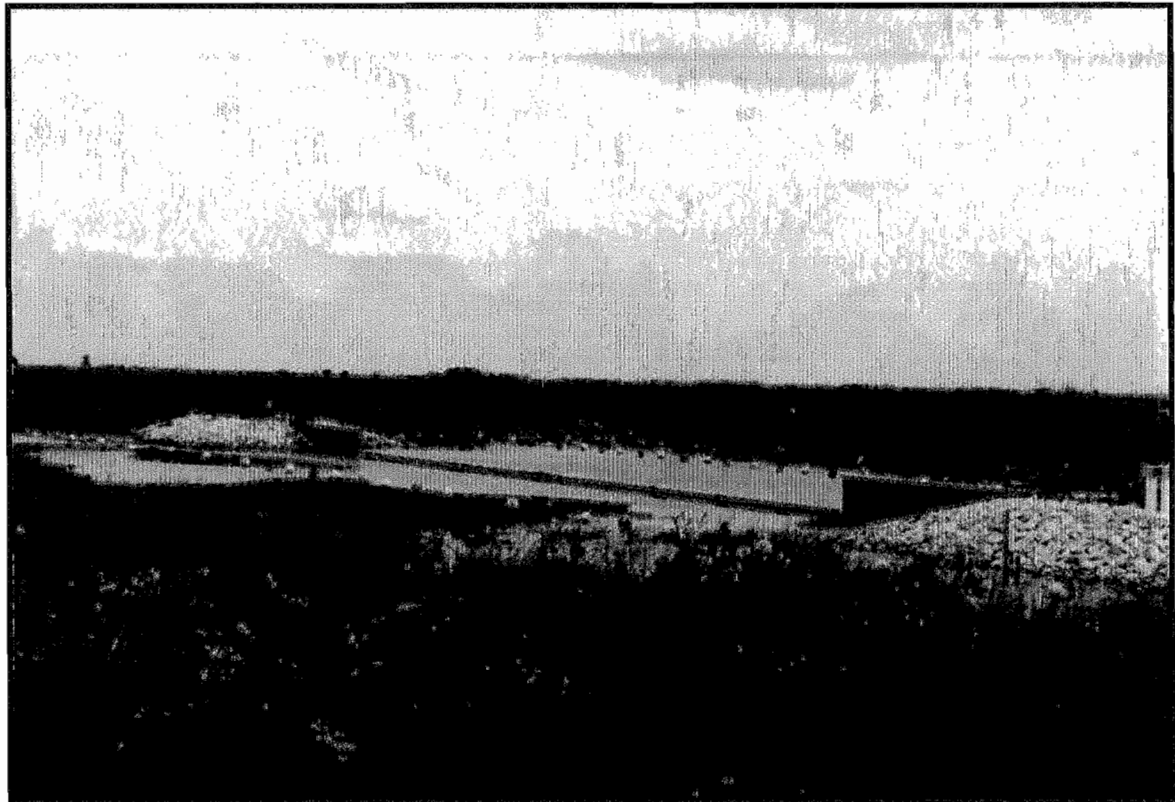
S-253 Weir, looking southeast from L-79.
