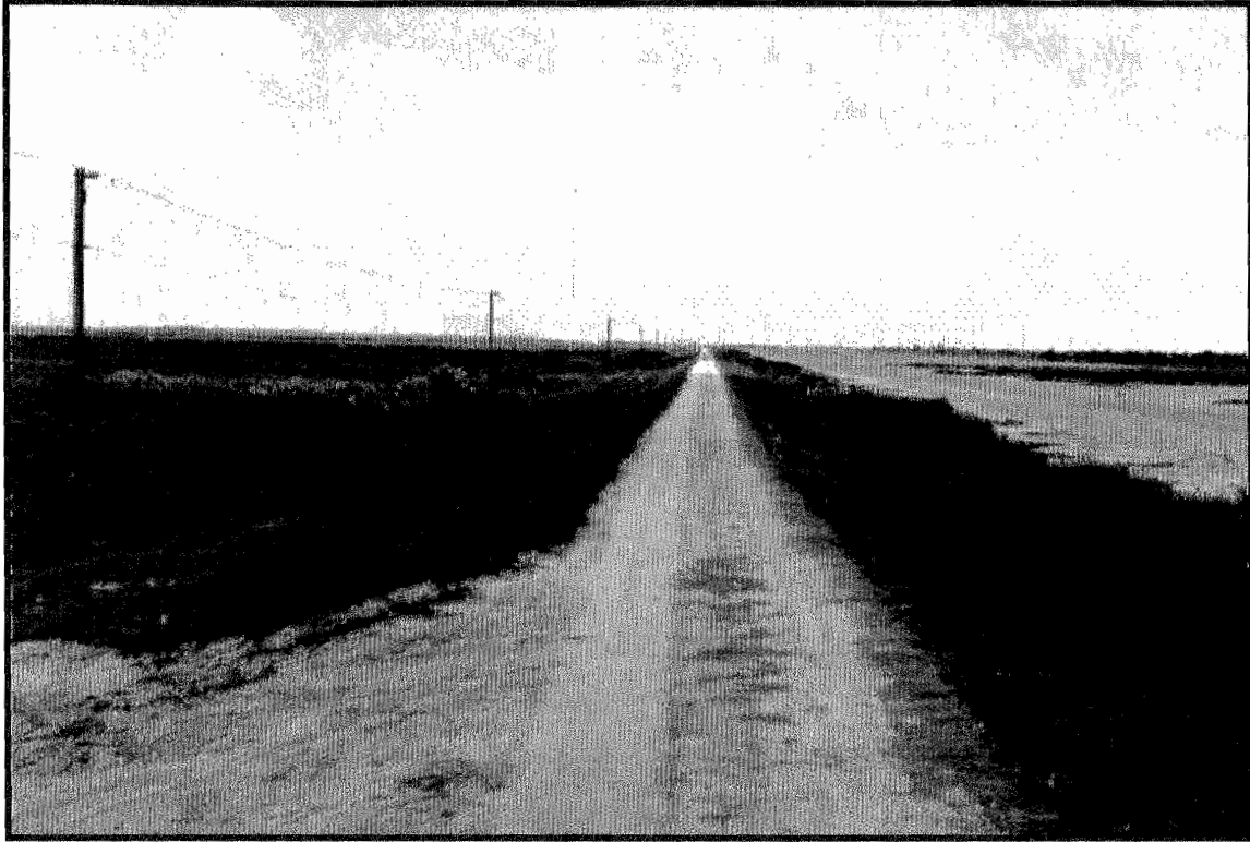
Levee-74-E, looking east from western end.
