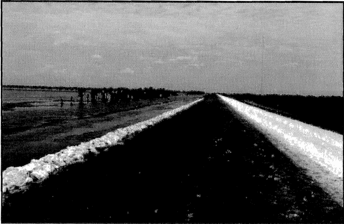
Levee-75, looking north, just south of S-96.
