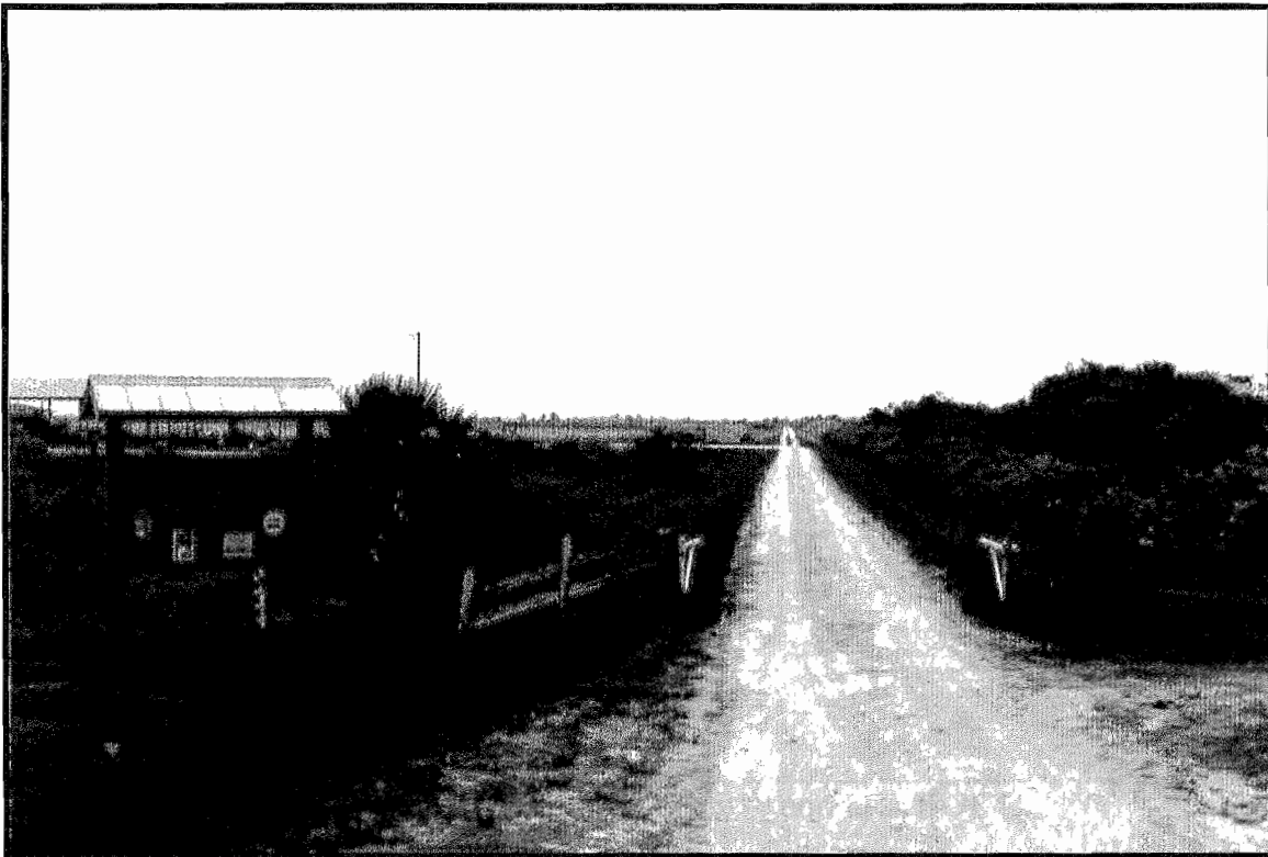
Levee 75-N, looking north at Fish and Game office entrance gate.
