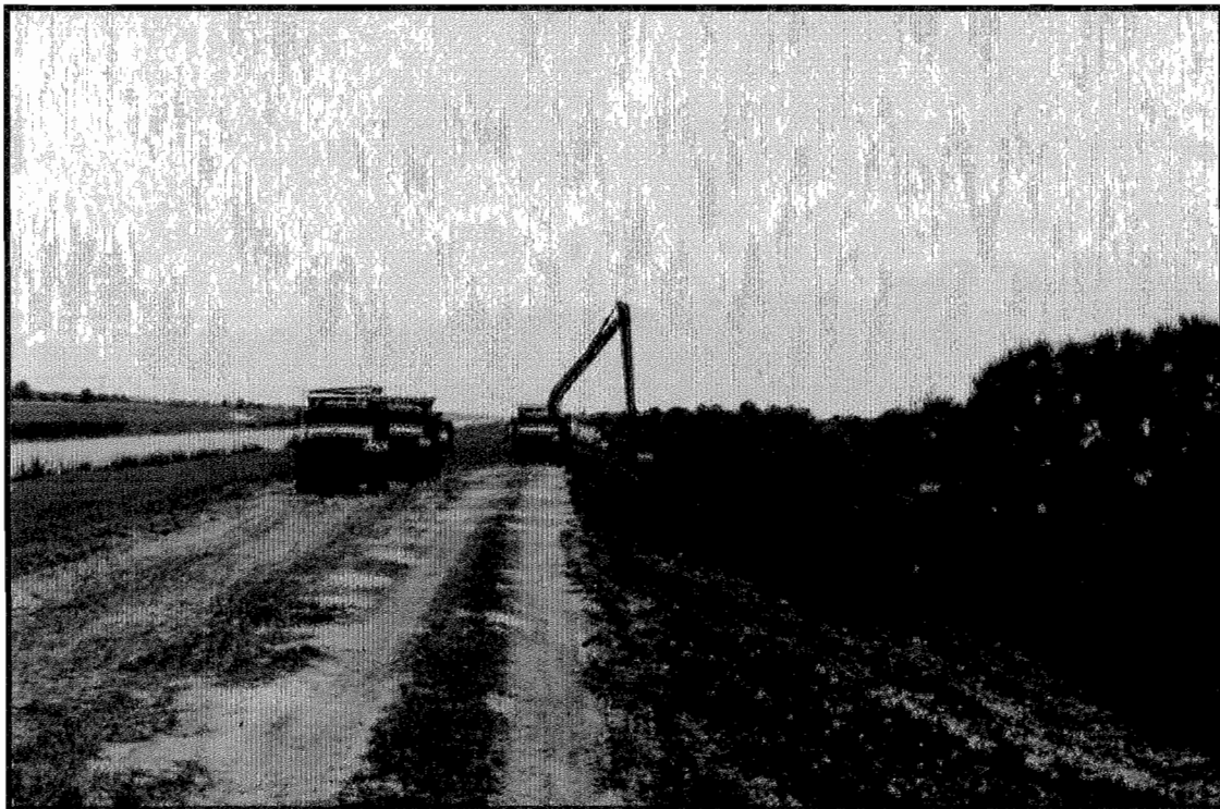
Levee-54, looking east on south side, east of S-96.
