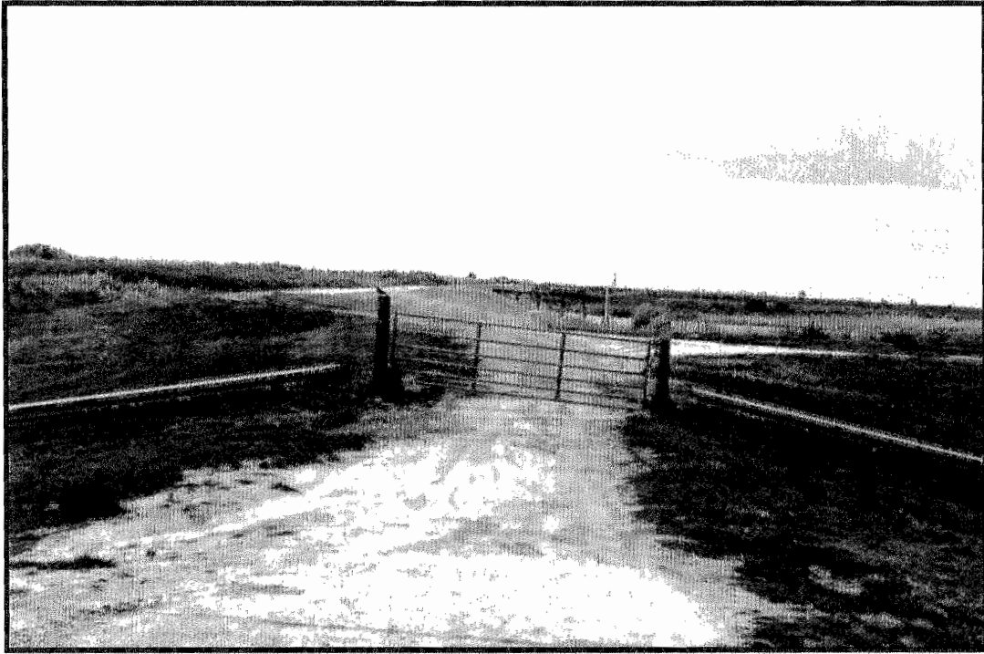
Levee-79, looking south from SR-60 entrance gate.
